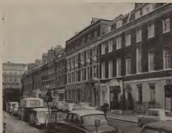
166 Percy Street. A terrace worthy of preservation.
